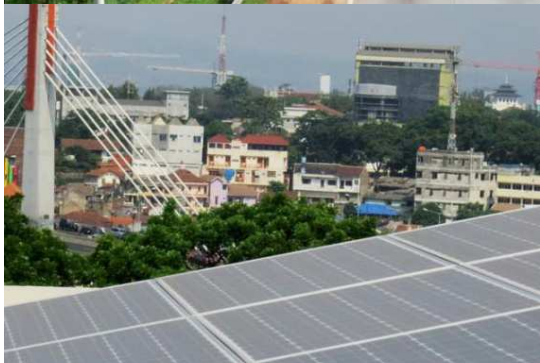
Roof Top Solar System
